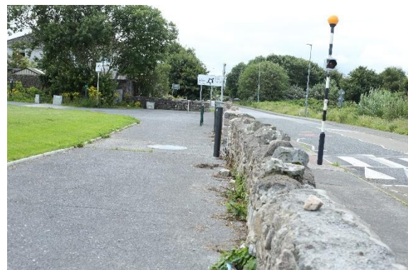
Plate 3-4: View of the existing active travel entrance and zebra crossing on the L-5000 road to the south of the site.
